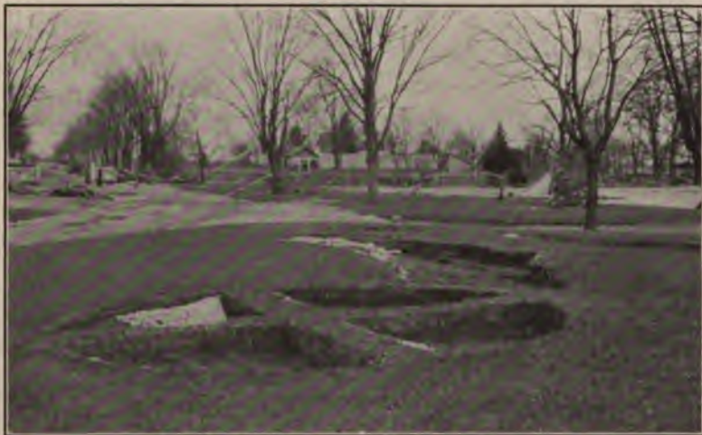
FIG. 33—This illustrates the value of sod in the prevention of erosion. Note the stones in the eroded flower bed that have been washed from the macadam roads.
